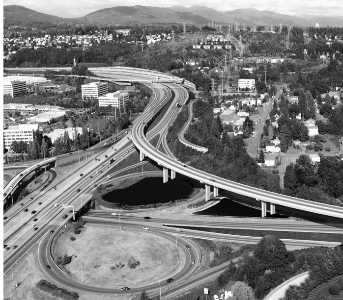
The future SR-167/I-405 HOV lane flyover
